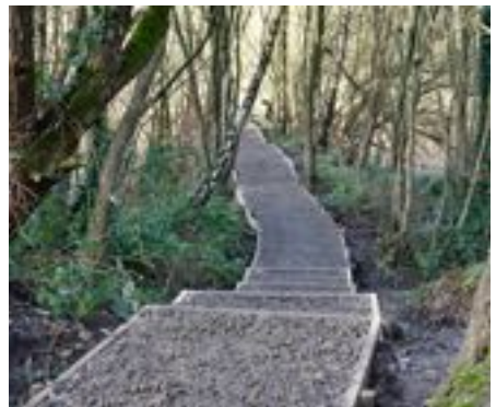
The new path & steps, built by contractors & Thursday working party 2019
