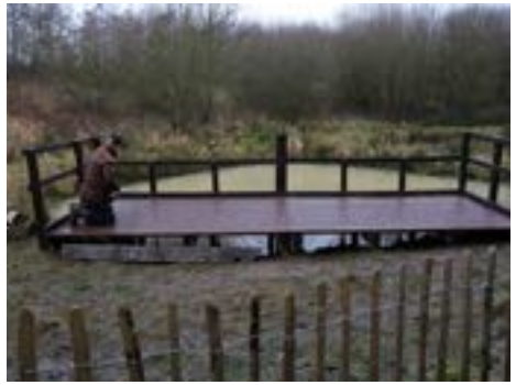
Putting the finishing touches to the pond dipping platform
