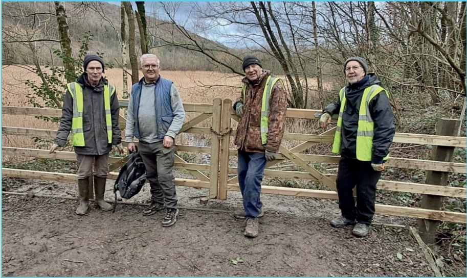
Proud volunteers having erected a new gate at the lagoon, again to prevent the spread of Crassula.
